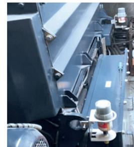
Automatic relubrication of generator bearing
