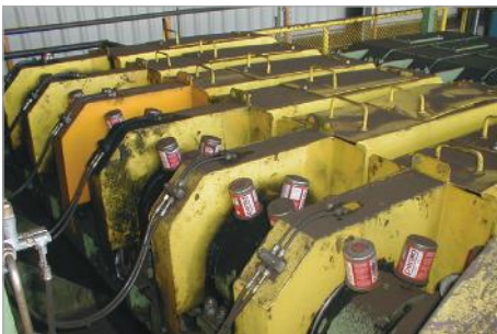
Lubrication of pillow block bearing on a drive shaft
