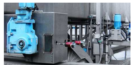
Wheel bearing lubrication at circular scraper
