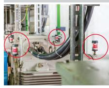
Bearing lubrication for electric motors
