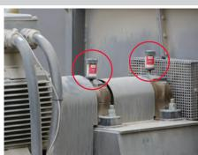
Roller bearing lubrication on the hot vertical bucket conveyor
