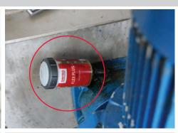
Bearing lubrication on a pump
