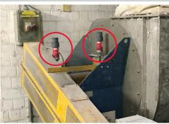
Lubrication of pillow block bearing on a fan
