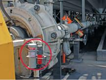
Bearing / seal lubrication on a pump
