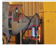
Bearing / seal lubrication on a pump
