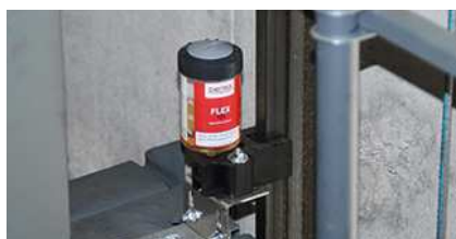
Lubrication of guide rails on passenger cabs
