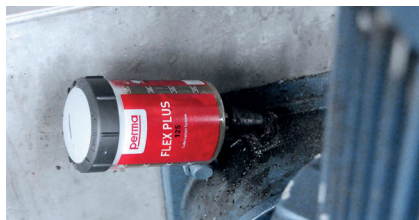
Bearing lubrication on a pump
