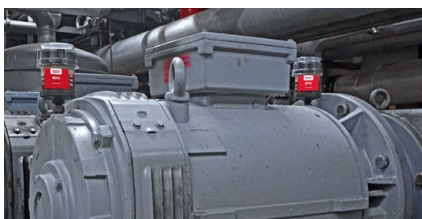
Electric motor lubrication on coolant compressors
