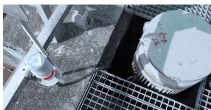
Bearing lubrication for electric motors
