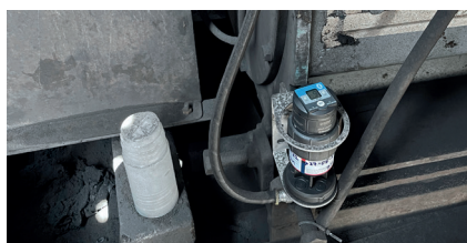
Bearing lubrication for electric motors
