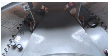
Blade bearing lubrication
