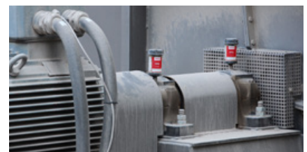
Pillow block lubrication on an exhauster
